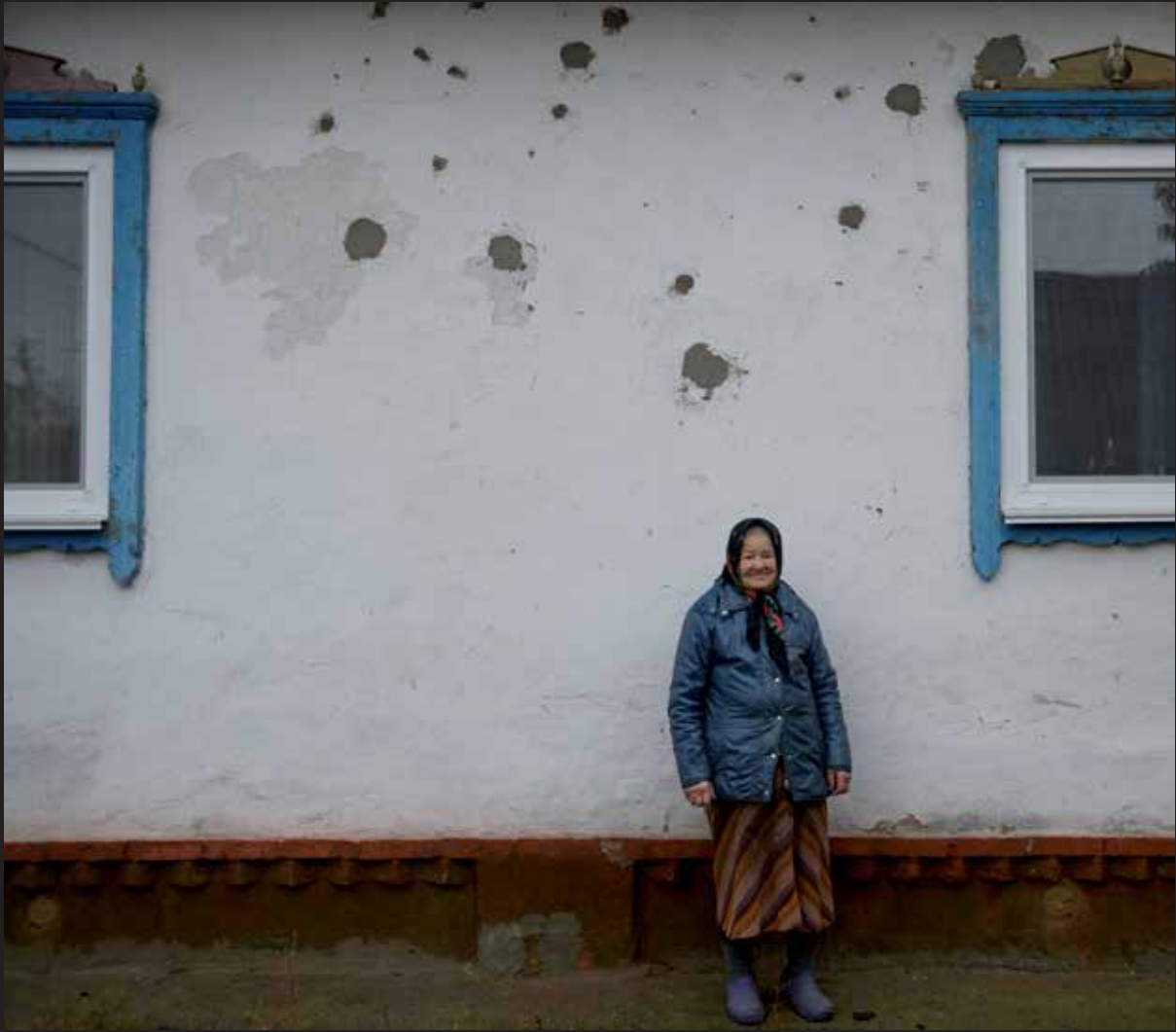
© ↑ Olha Kot in front of her home which was heavily damaged during attacks in Chernihiv, Ukraine. © Amnesty International
